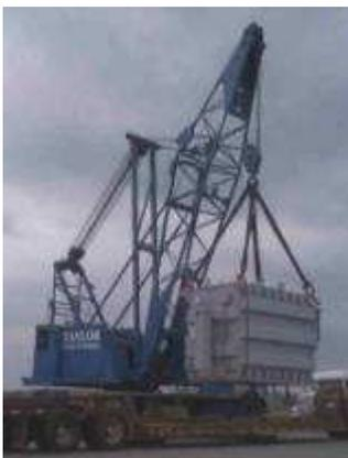
**A new 25 MVA transformer for the Industrial Park Substation is unloaded – Spring 2000.**
