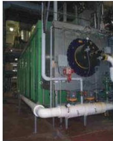
*220,000 lbs/hr Nebraska Boiler installed at the power plant in 1997.*
